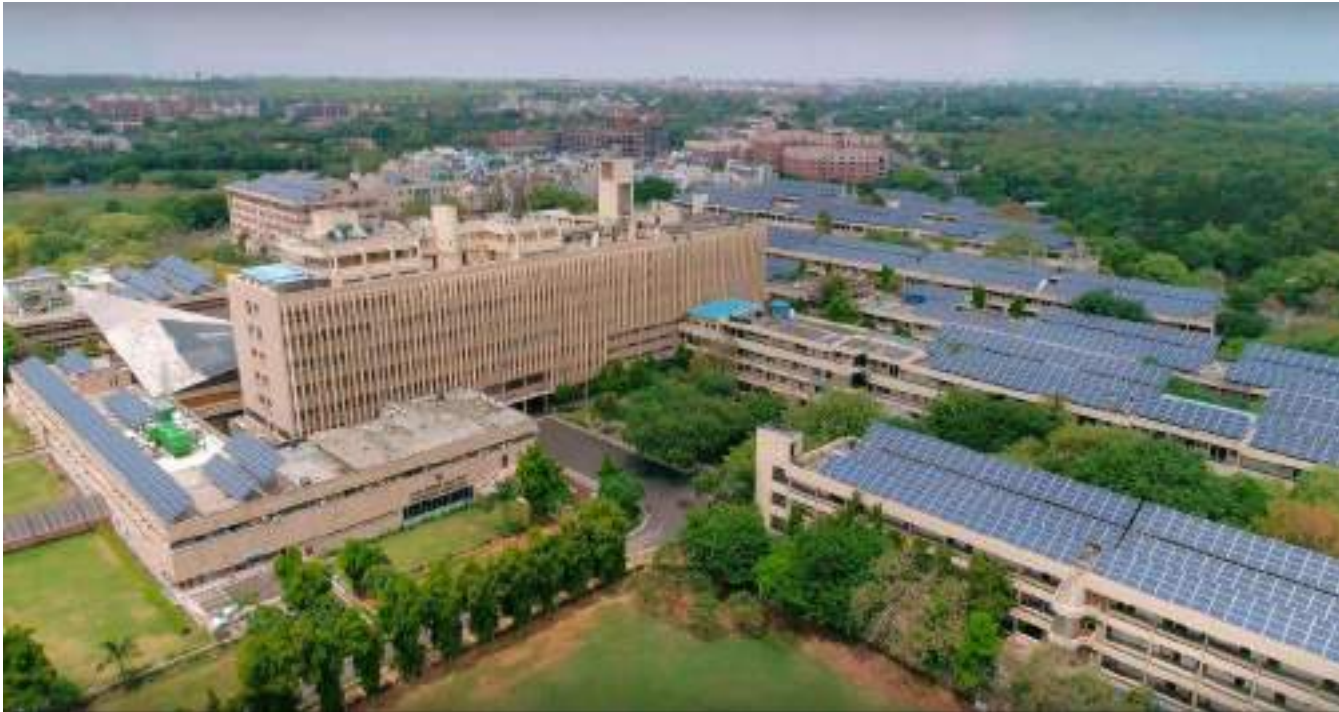
2.8 MWp Solar PV on campus rooftop, 2 MW hydropower purchase
