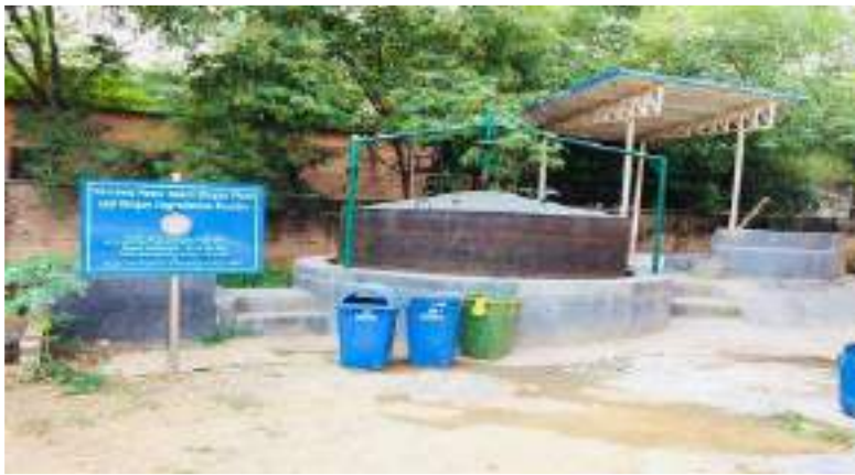
Anaerobic digester using kitchen waste
